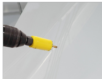
[Figure 13] Drill a 22 mm hole for the feedthrough of cables
